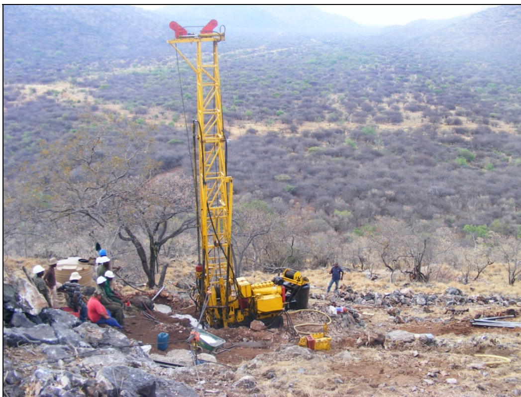
The drill rig in position on the first drill pad at Kaskara.
